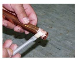
4. Apply the soldering flux on the pipe
