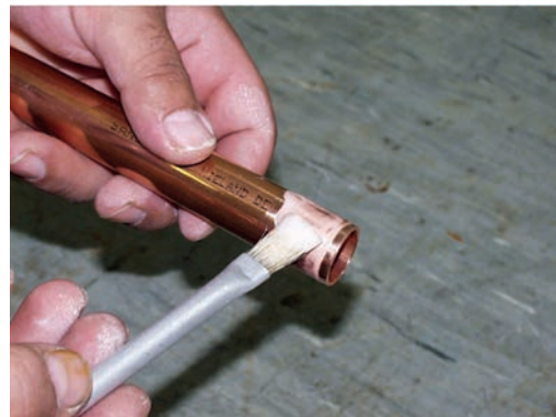
4. Apply the soldering flux on the pipe
